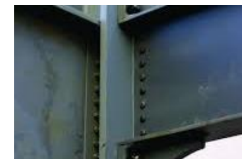
steel beam-column connections
