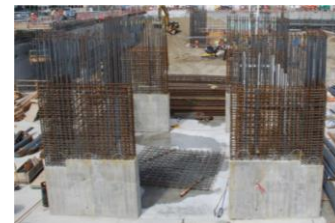
reinforced concrete walls
