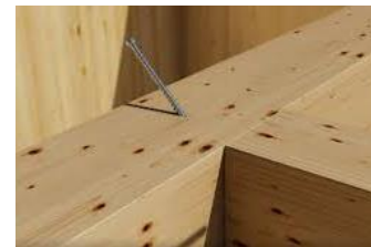
toe-screwed wood connections
